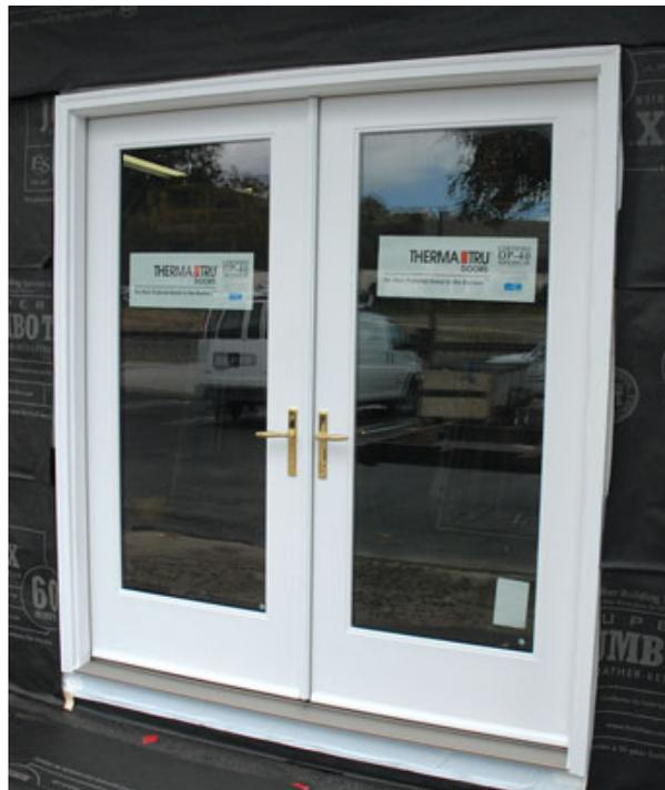
**Figure 8.** The top flashing laps over the upper nailing flange and is installed after the door is in place (above). Housewrap can be installed either before or after the door unit (left).
